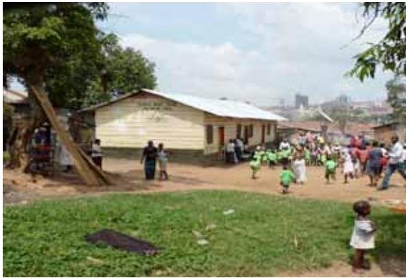
Like most schools in the slums of Kampala, Nalinya Bright Future primary school is run by teachers without any public funding. The renovation, funded by Foundation Croix du Sud, cost € 3000.
